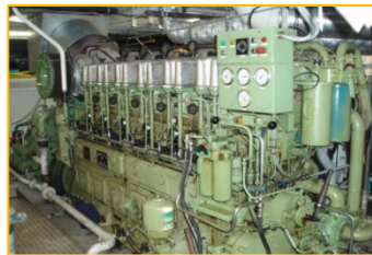
MS Aarburg • Main engine: ABC MDZC-166 A • 1.325 kW • Container Ship • 135 m • 3.297 to.
