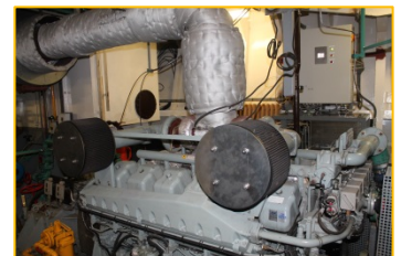
MS Aarburg • Main engine: ABC MDZC-166 A • 1.325 kW • Container Ship • 135 m • 3.297 to.
